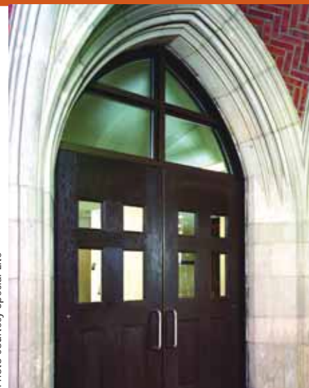
Aluminum/composite hybrid flush doors can be made with plastic face sheets with a wood grain texture.
