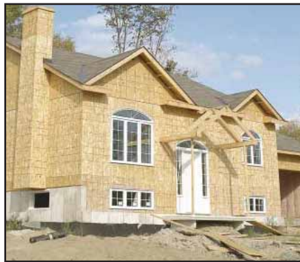
OSB panels meet the requirements of a wide variety of building codes.
