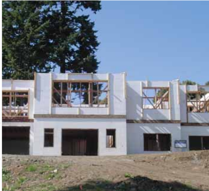
SIPs help reduce air infiltration in comparison to wall assemblies made of traditional materials.
