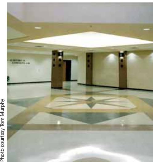
Thin-set terrazzo, a composite material, tends to crack less than traditional flooring products.
