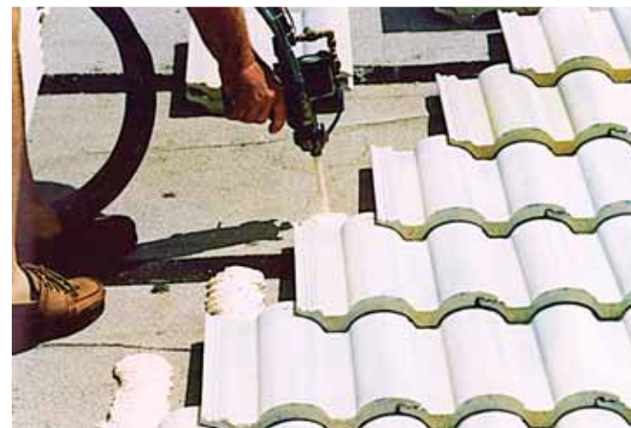
Bound together with polymer adhesives, composite roofing shingles provide long service life.
